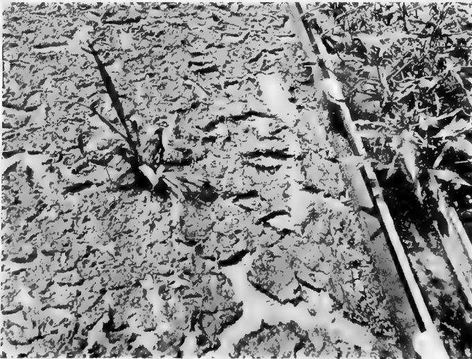
Fig. 49.—Dried sediment on the surface of a sand filter of a sewage disposal plant.
